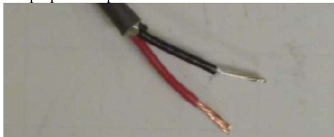
Figure 47- Shield wire end prep completed
