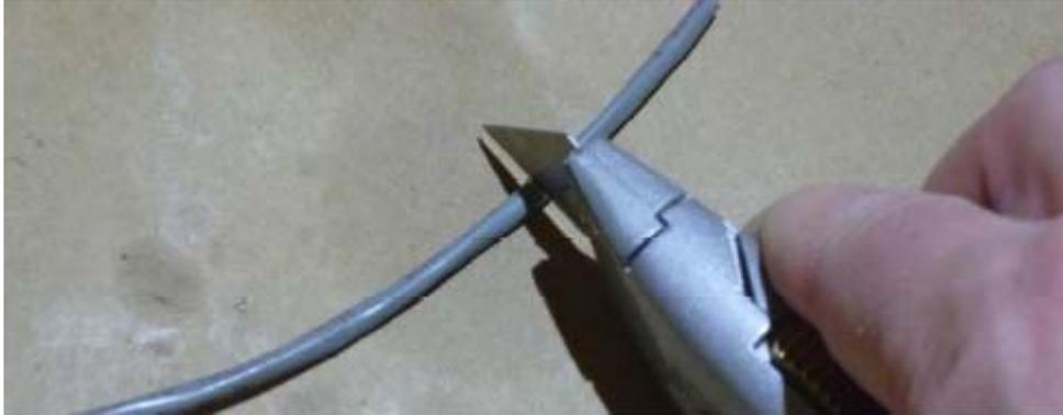
2. Use a utility knife with a new, sharp blade to cut the plastic jacket of the shielded cable 1" back from the end. Hold the blade perpendicular to the cable, and draw it across the cable lightly as you rotate the cable along its long dimension. This creates a scored line through the plastic jacket. With a sharp blade, not much pressure is needed. You may need a bit of practice to get the feel.
